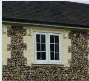
Casement window with flint walling
